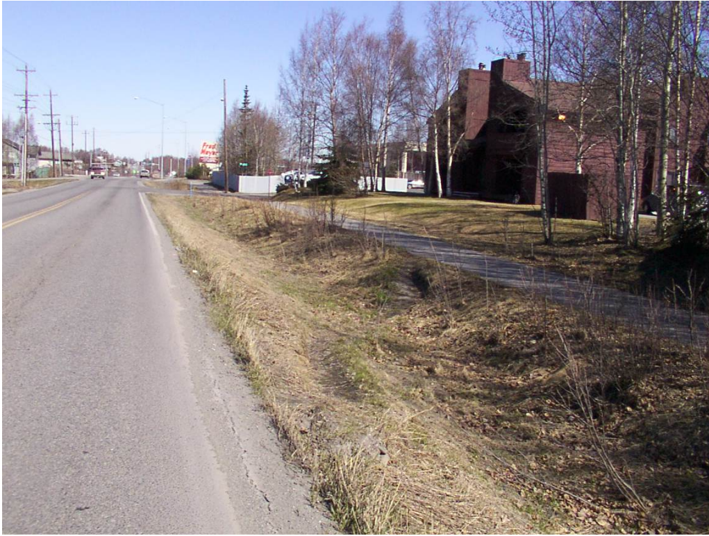
Detached pathway on East side of Victor Road.
