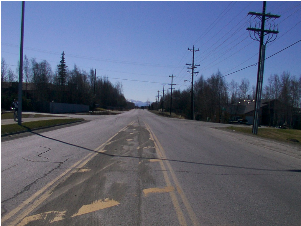
Many utilities are present in the Victor Road corridor.
