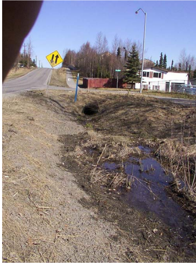
Drainage is conveyed by ditches and culvert system.
