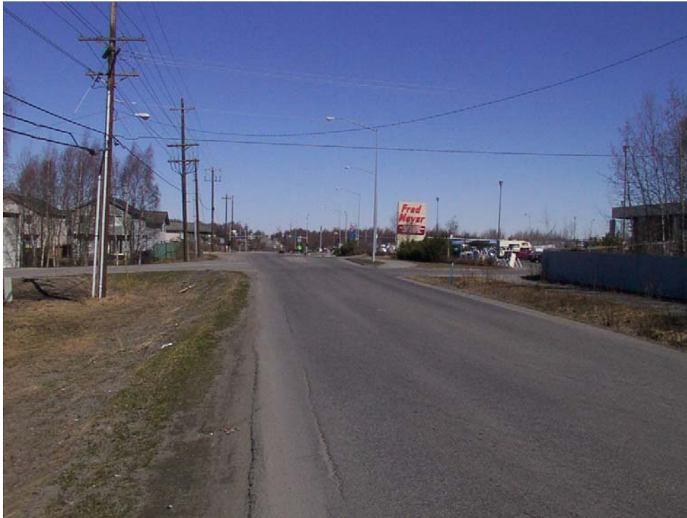
Road with narrow unpaved shoulders.
