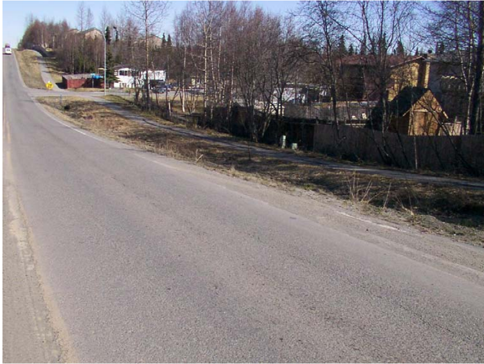
The existing road is higher than the surrounding ground and ditches are adjacent to the travel lanes.
