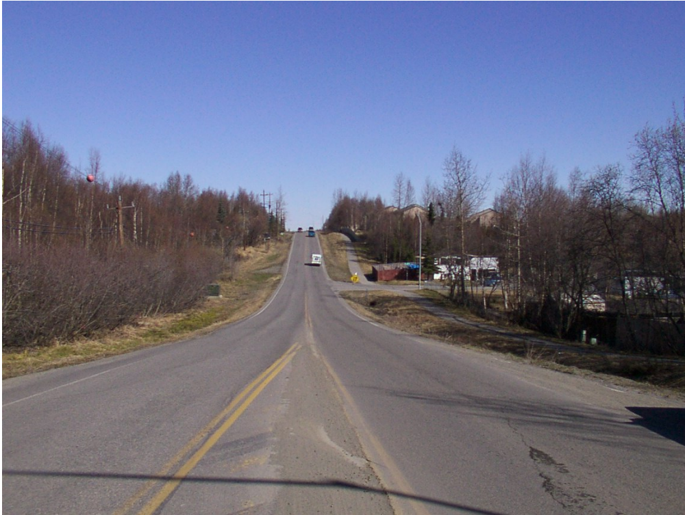
Existing Victor Road has narrow lanes and steep grades.
